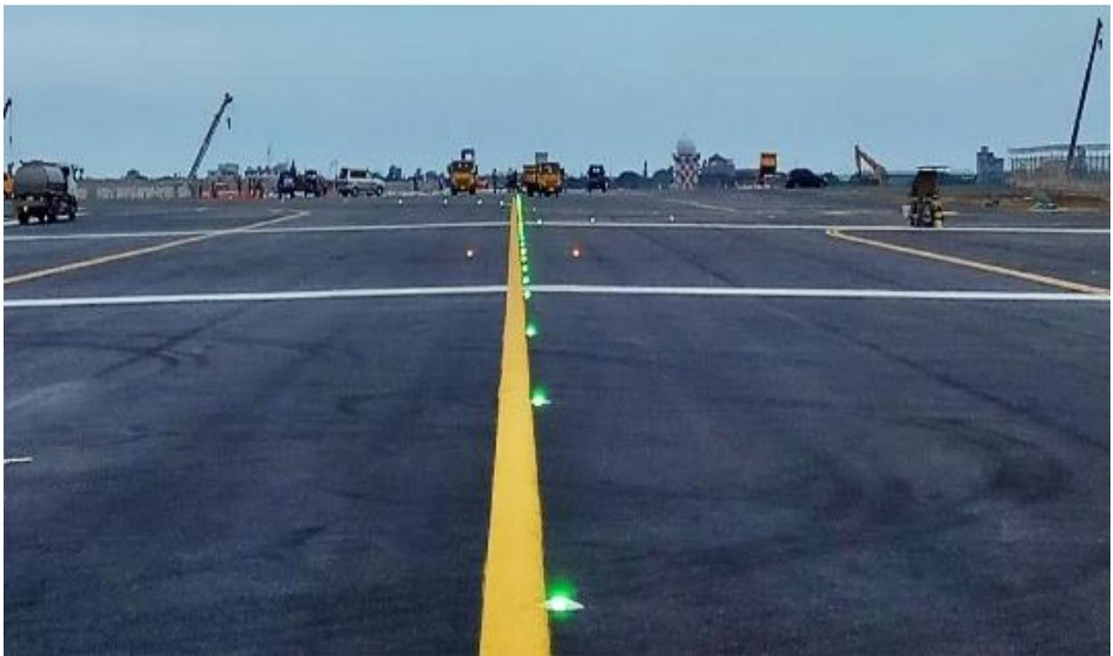
W2滑行道南段助導航燈光系統供電及測試情形
